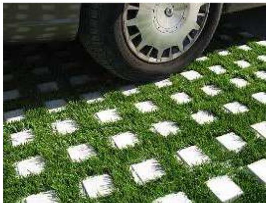
*A range of paving details, clockwise from top left: brushed finished concrete and permeable block paving; natural stone kerb and sett threshold and bituminous macadam detail; reinforced grass using 'Checker Block' concrete modular product; panels of brushed finished concrete within lawn, showing integration of paving and soft landscape.*
